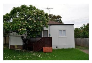
The rear of the house appears to be clad in asbestos containing "Fibrolite" panelling which was widely used for such elements in the late 1920s and up until the 1970s.
