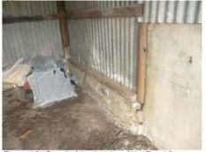
Figure 10. Detail of the interior of the Feed Store showing the condition of part of the concrete footing and dwarf wall.
