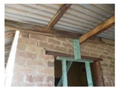
Figure 6. Door opening between the Equipment Room and Feed Store to be reconstructed.
