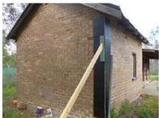
Figure 5. Temporary repair to the NE comer of the Cool Room
