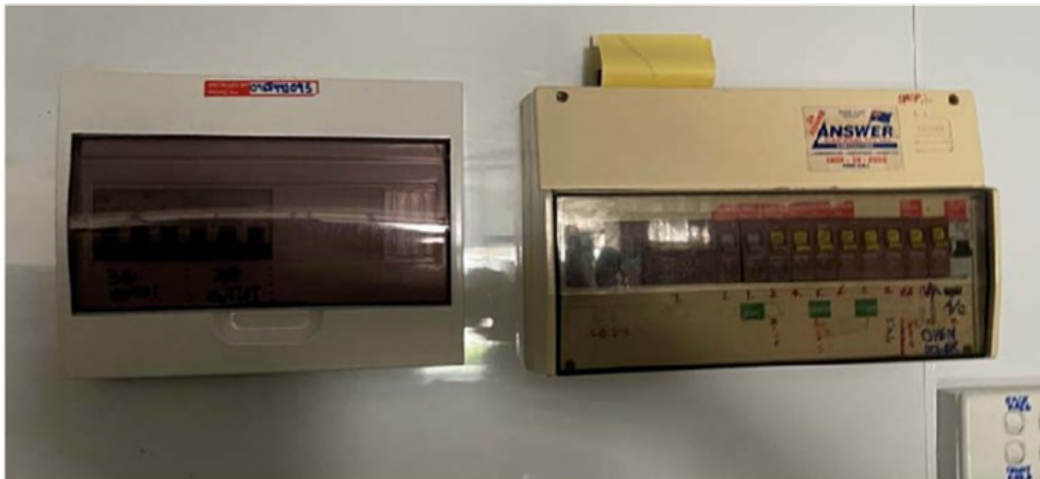
Figure 1 – Existing Shop 2 Switchboard
