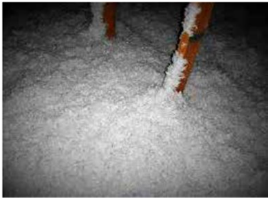
Loose fill ceiling insulation
