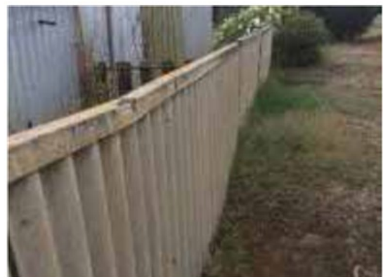
Corrugated asbestos cement sheeting used as a fence in local park
