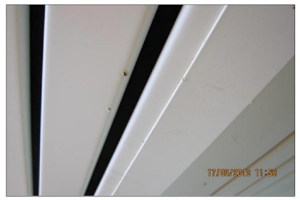
PHOTO 1: PITTING CORROSION TO INDOOR CEILING
