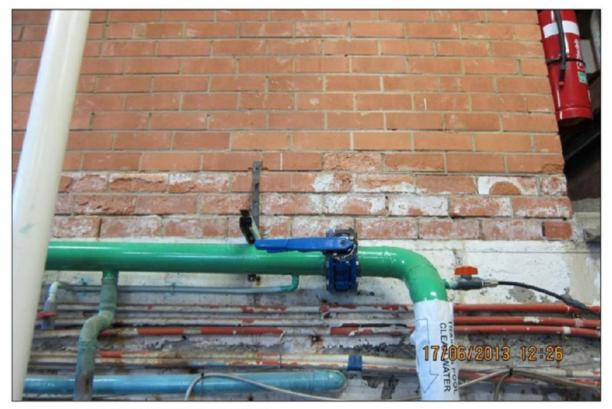
PHOTO 8: SULPHATE ATTACK TO MASONRY
