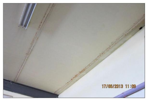
PHOTO 5: CORROSION TO CEILING CHANELS
