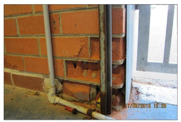
PHOTO 7: SULPHATE ATTACK TO MASONRY
