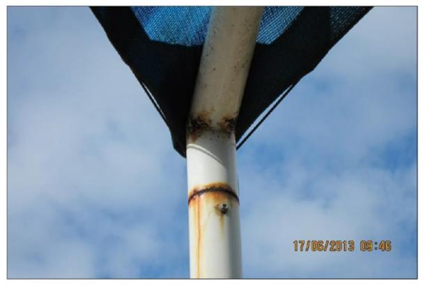
**PHOTO 4: SHADE STRUCTURE CORROSION**
