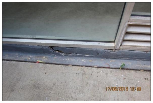
PHOTO 4: CRACKING TO CONCRETE HOB
