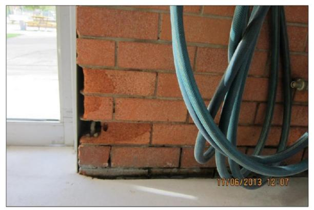
PHOTO 3: SULPHATE ATTACK TO MASONRY
