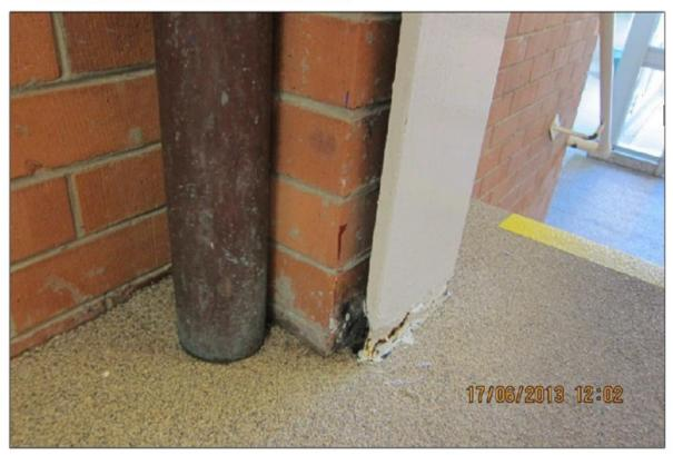
PHOTO 2: CORROSION TO STEEL COLUMN
