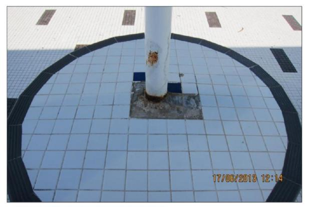
PHOTO 5: CORROSION TO SHADE STRUCTURE SUPPORT
