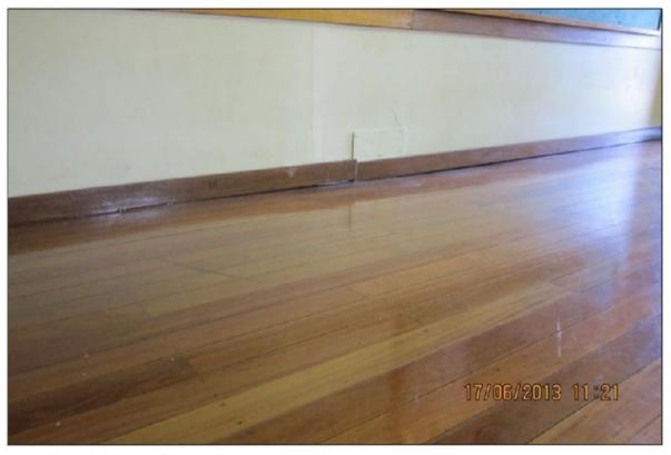
PHOTO 6: DEFLECTION OF BEARS AND FLOOR JOIST
