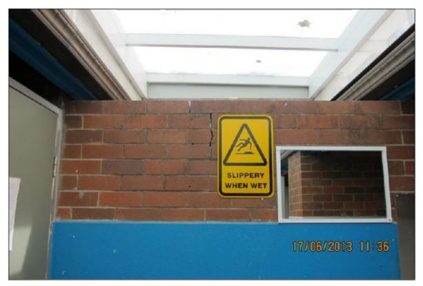
PHOTO 9: MASONRY CRACK MALE TOILETS
