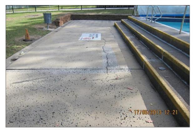
PHOTO 9: PAVEMENT CRACKING
