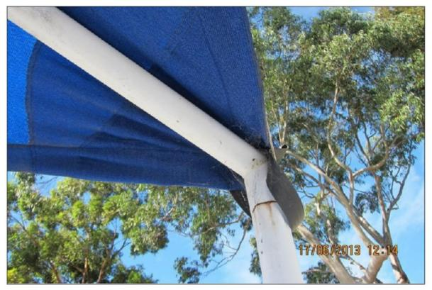
PHOTO 6: CORROSION TO SHADE STRUCTURE
