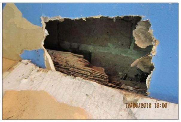
PHOTO 10: TERMITE DAMAGE
