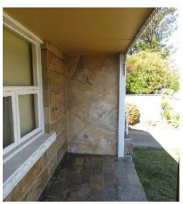
**Figure 4.4** View south at front verandah with lowered ceiling, c1950s tiling and infill to end.
