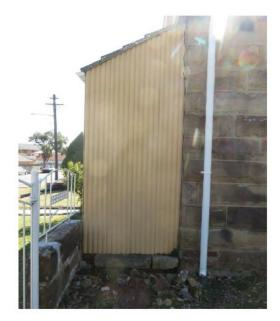
**Figure 4.11** Southern end of verandah showing corrugated metal backing to enclosed verandah.
