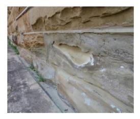
**Figure 4.15** Detail of sandstone blocks along northern elevation showing signs of deterioration and spalling from salt attack/rising damp.
