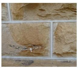
**Figure 4.16** Detail of sandstone blocks showing concrete repointing work.
