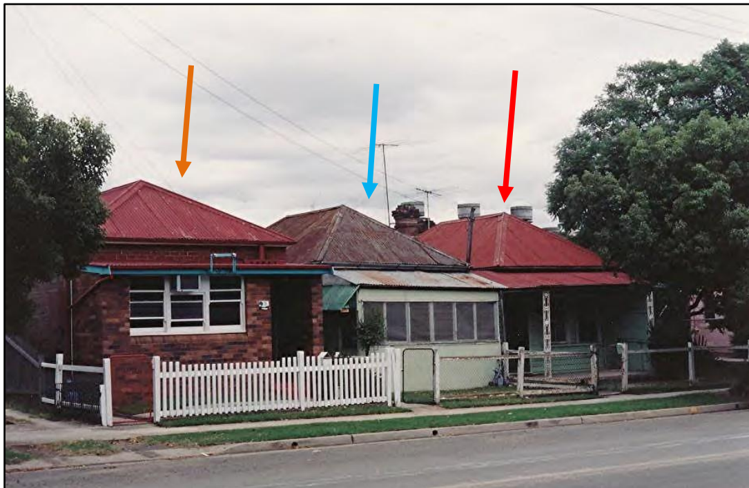
Figure 34. 1992 image of the three properties comprising the original "William Street Cottages Group". The subject site (indicated by red arrow) still displays original or early features at this time, including roofing, chimneys, front fence, and verandah posts. The neighbour cottage at no. 8 William St (indicated by blue arrow) is still extant at this time, although the original cottage at 6 William St (indicated by orange arrow) had been demolished (Source: City of Parramatta, 8-10 William Street, Heritage Study , 1992).
