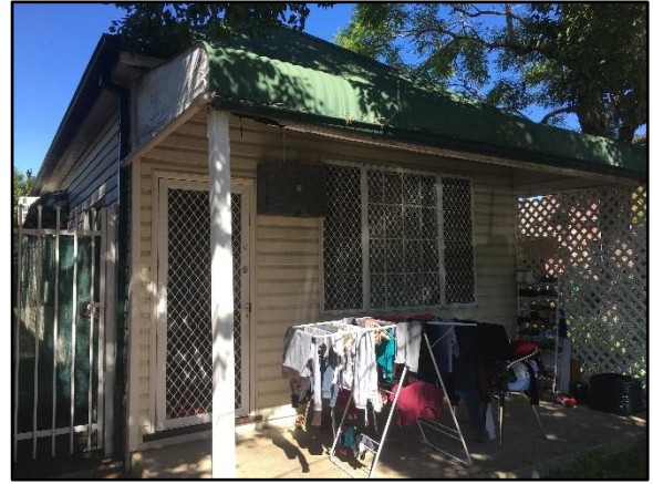
Figure 9. Front veranda displaying bullnose roof, turned timber post, and lattice on western side.
