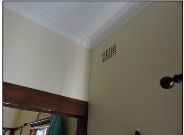
Figure 27. Living room ceiling.
