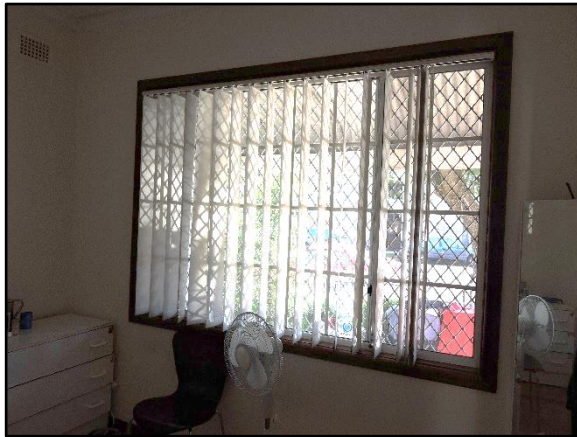
Figure 20. Fenestration in front bedroom.
