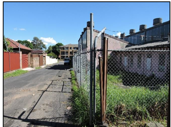
Figure 17. View facing west from access lane at rear of property.
