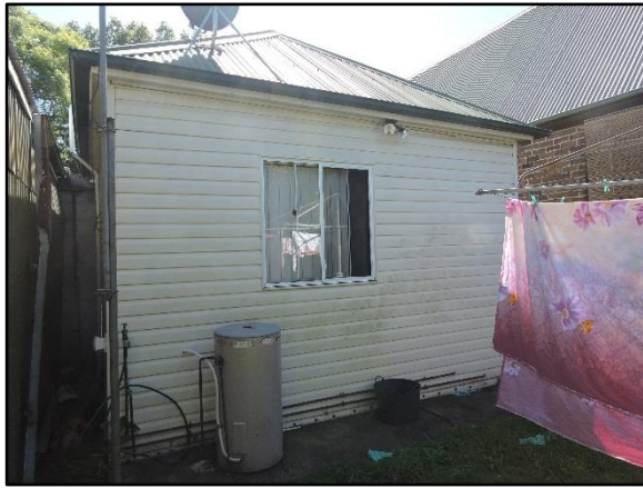
Figure 14. Rear elevation of dwelling.
