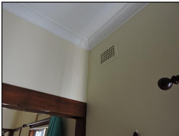
Figure 24. Ceiling in hallway.
