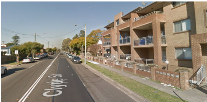
Existing higher density residential on Clyde Street
