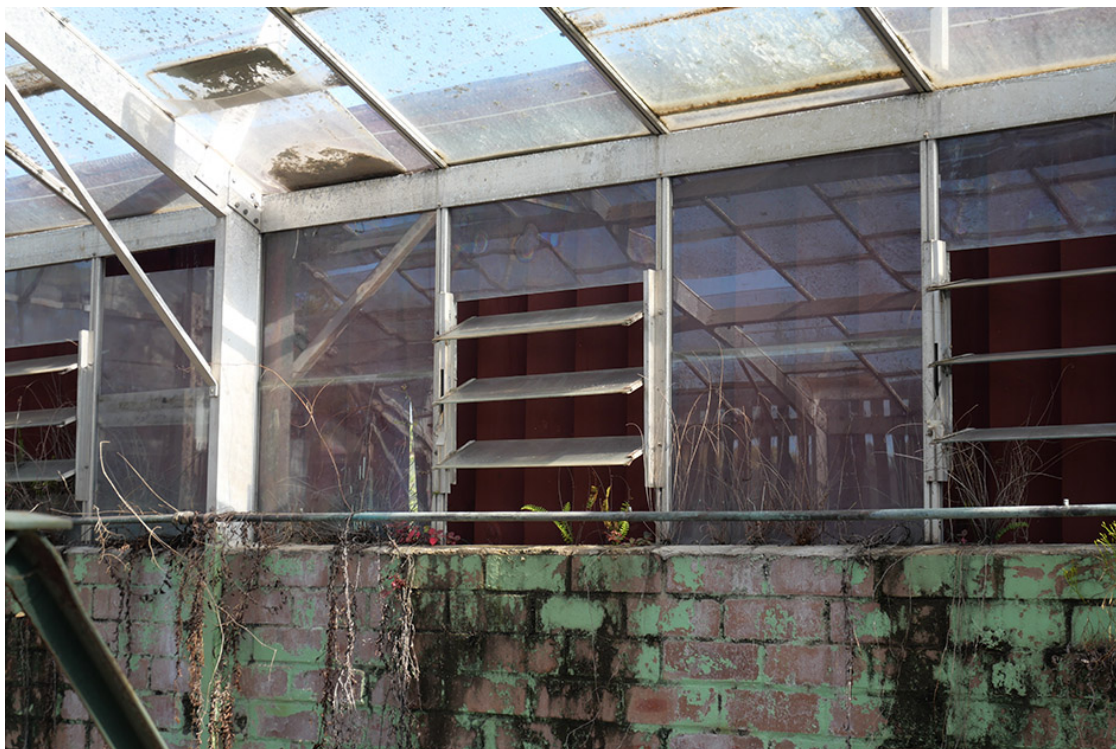
Detail of brickwork, fixed glazing and glass louvres to glasshouse wall, taken from interior of glasshouse
