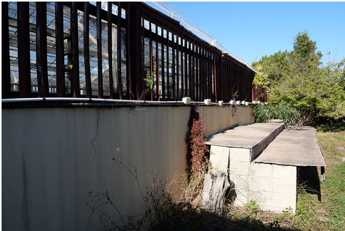
View along the western exterior wall of the glasshouse, with timber external vertical slats
