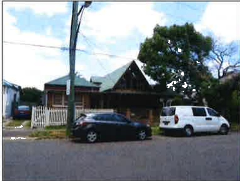
Figure 3: No.6 and No.8 William Street
