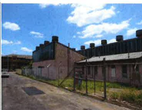
Figure 6: View west along laneway of rear of No. 12 William Street
