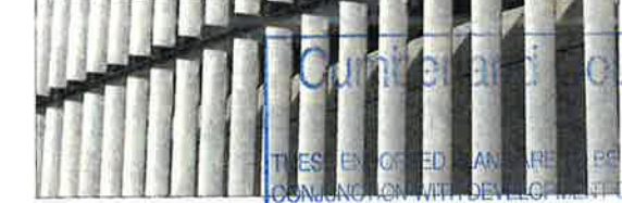
8. 350x50 MM POWDER COATED ALUMINIUM FACADE LOUVRES
